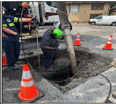
July 31 st – Excavator Crew – Little Falls
