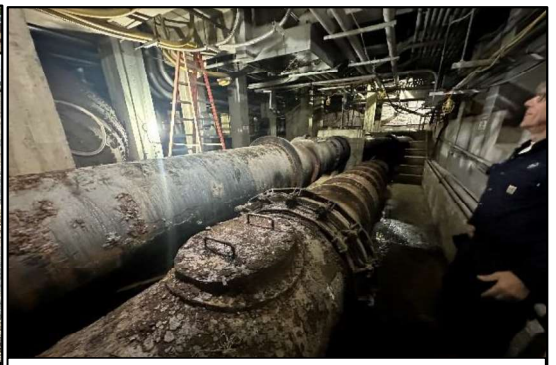
November 18 th – Electrical Work – Main PS Basement
